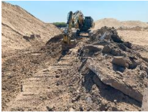
Removal of Rubble from the dunes (2025)
