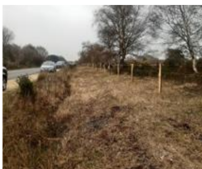
Installing perimeter fence
