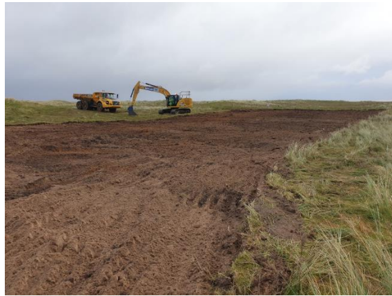
Turf and soil stripping
