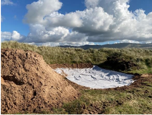
Pond being installed at Eskmeals, Cumbria
