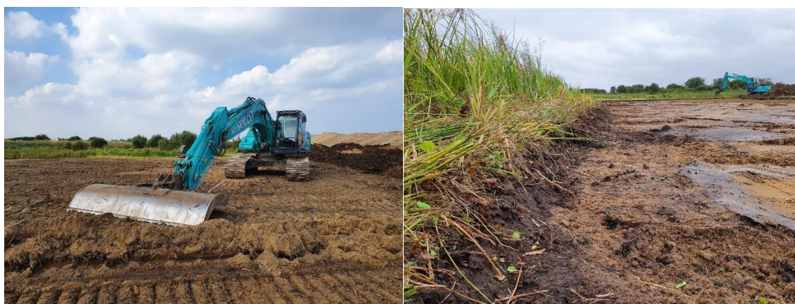
Turf stripping 1ha of the freshwater marsh at Saltfleetby-Theddlethorpe NNR
