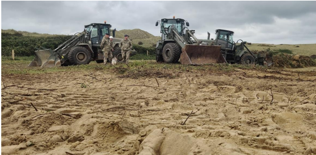
Military personnel assisting with increasing the amount of mobile sand at Penhale.
