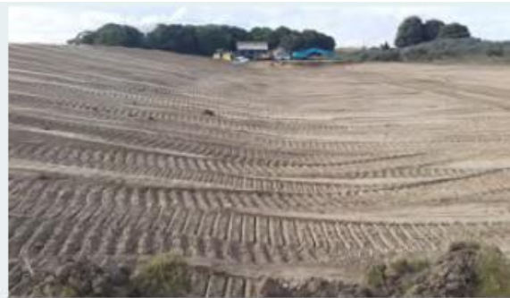
2021 during construction. Photo Lincolnshire Wildlife Trust
