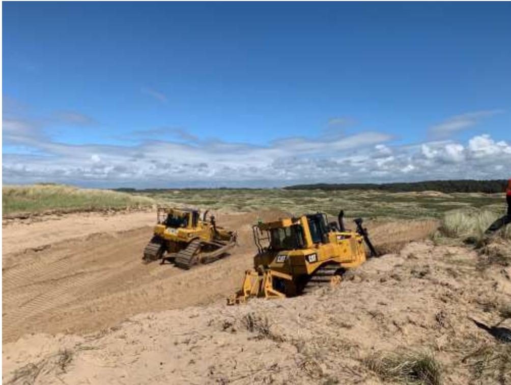
Photo 7: Notch work underway in May 2022
