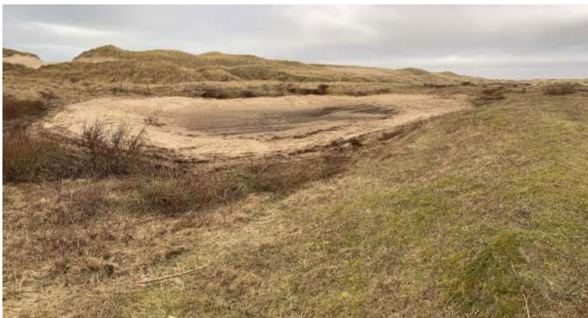
Photo 12: Completed dune slack scrape in February 2023
